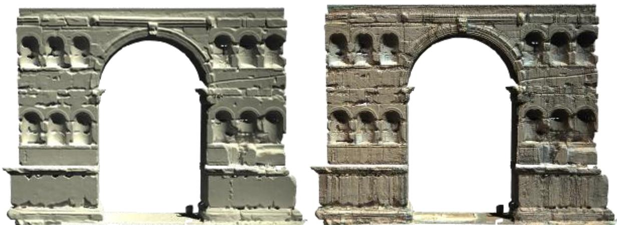
*Fig. 3 Arco di Giano in Rome. Three-dimensional model with and without the photographic texture*
