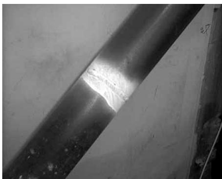
Figure 13 Welding between tubular profiles
