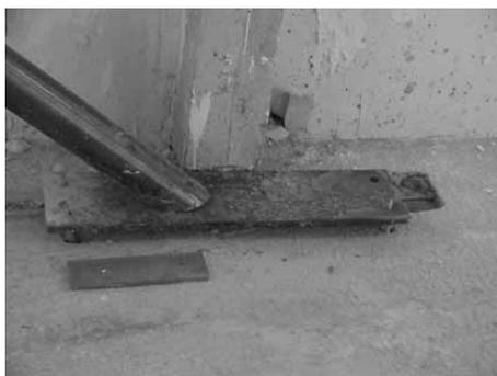
Figure 15 Bottom steel plate for anchoring
