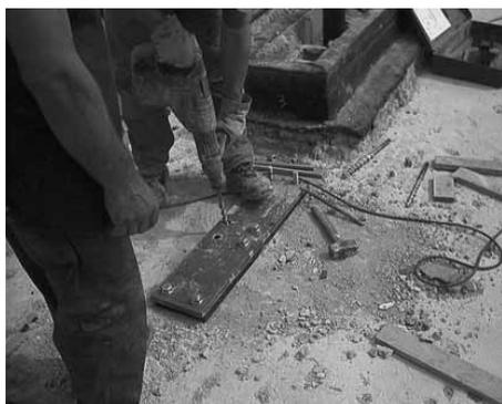
Figure 16 Anchoring operations to the existing floor
