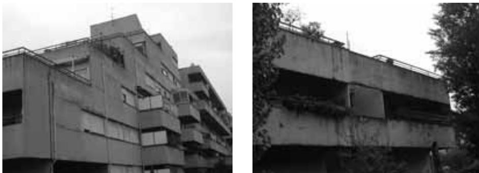
Figure 4-5. Decay of the façades due to atmospheric agents
