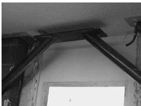
Figure 14 Top steel plate for anchoring
