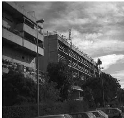
Figure 2-3. The structure formed by parallel concrete walls is visible in the modularity of the façade
